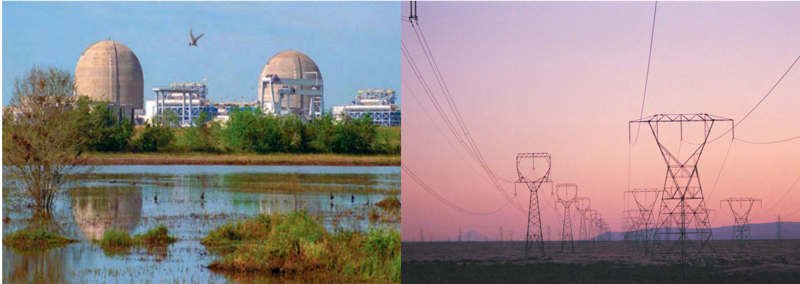
Figure 1 The South Texas Nuclear Project and a Bulk Transmission Corridor
