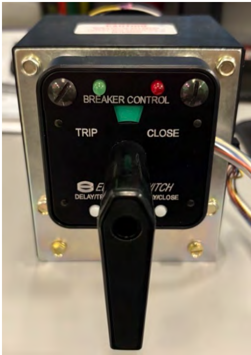
Fig. 6 Circuit Breaker Time-Delay Control Switch
