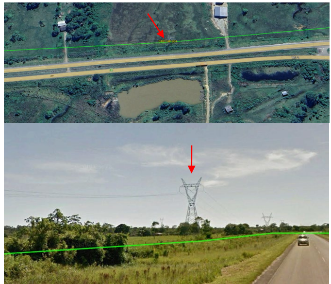
Fig. 39. Location of Tower T-034 (utility KMZ route files).
