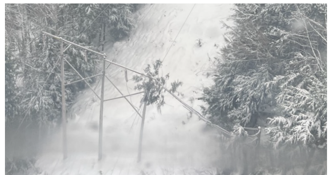
Fig. 10. A tree contact was the cause of the fault shown in Fig. 9 (photograph and fault records courtesy of Puget Sound Energy).
