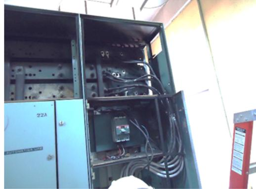
Figure 2 MCC Damaged in the 2012 Arc-Flash Event
