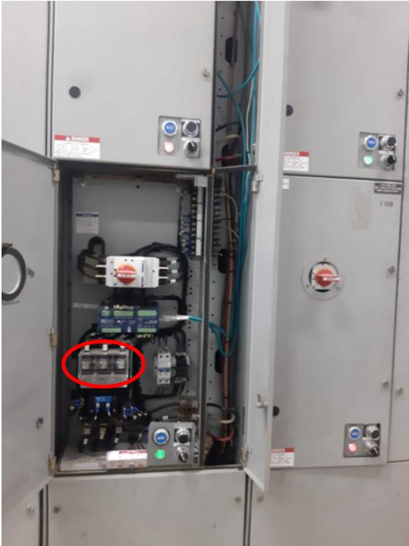
Figure 10 MCC Bucket With Installed Contact Cover
