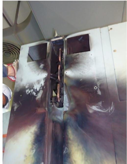
Figure 3 Horizontal Busbar of the MCC
