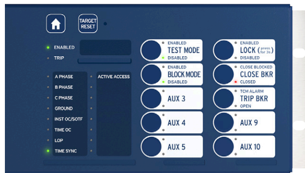
Figure 7 Status and Trip Target LEDs
