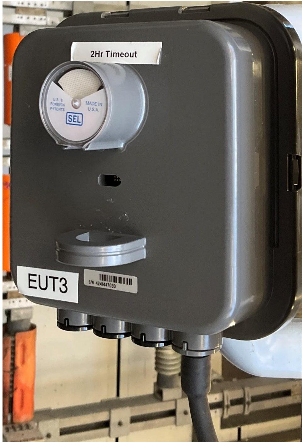
Figure C-3: Tested SEL-8317 LINAM® UGFI FCI unit.
