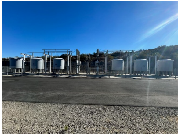
Fig. 6. SDG&E Bus Reactor Project Field Installation Example
