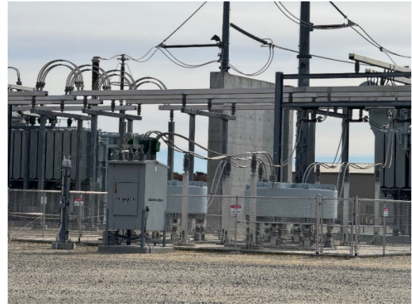
Fig. 10. Tertiary Reactor Installation Example
