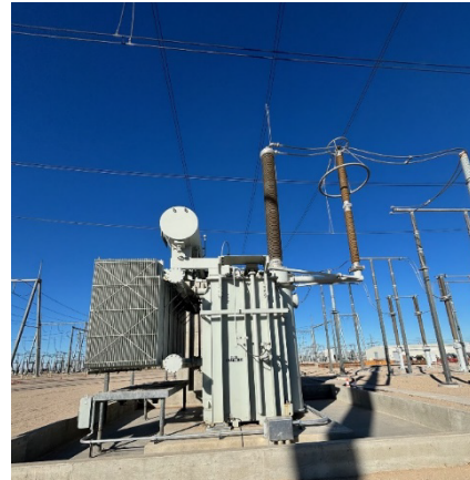
Fig. 16. Line Reactor Installation Example
