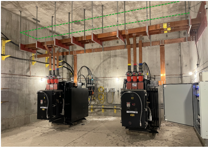
Fig. 15. Loop sensor installation in 480 V vault.
