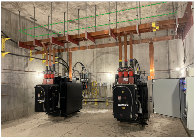
Fig. 15. Loop sensor installation in 480 V vault.
