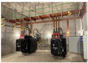
Fig. 15. Loop sensor installation in 480 V vault.
