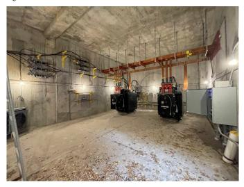
Fig. 7. Inside a large 480 V network vault.
