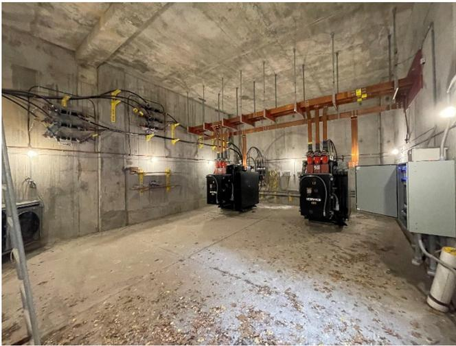
Fig. 7. Inside a large 480 V network vault.
