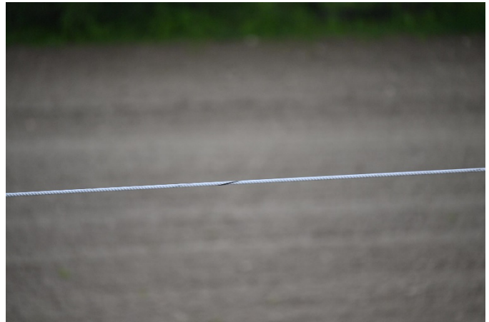
Fig. 14. A burn mark identified by the aerial patrol crew on the shield wire at the reported location.
