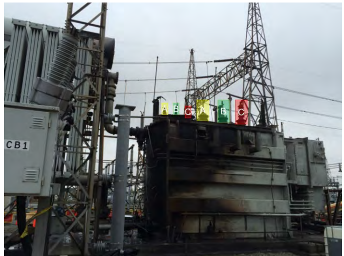
Fig. 9. Transformer damaged by the blaze.
