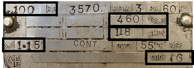
Fig. 17 Motor Nameplate for Example 2
