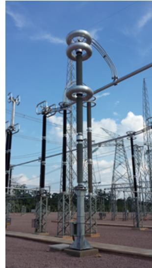
Fig. 9. The coupling capacitor at Araraquara Substation.
