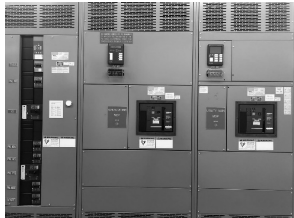
Fig. 1 Typical Service Entrance With Multiple Sources
