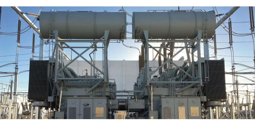
Protect and control PSTs, also known as phase-angle regulating (PAR) transformers, with purpose-engineered solutions.
