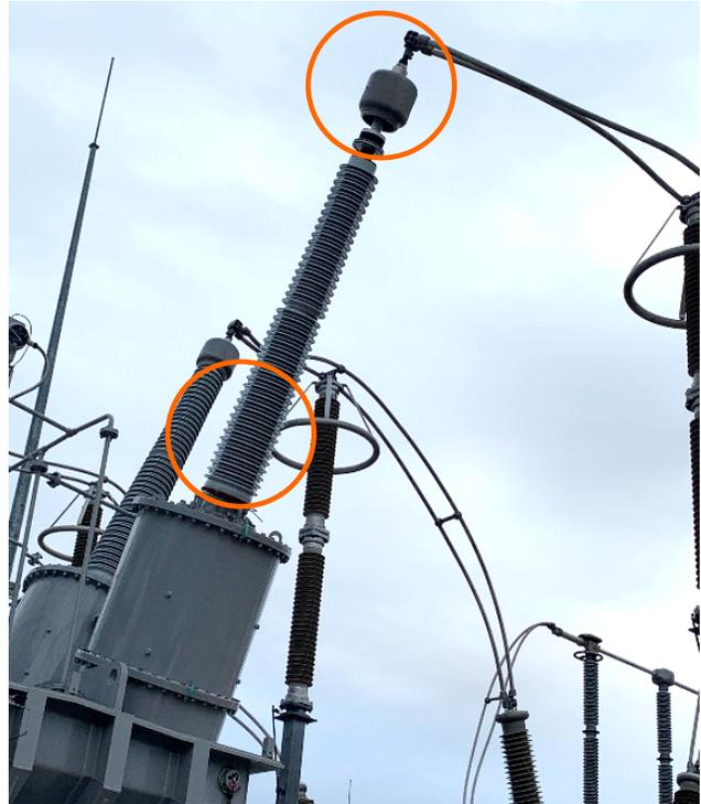
Fig. 23. Damaged reactor bushing at Romney.
