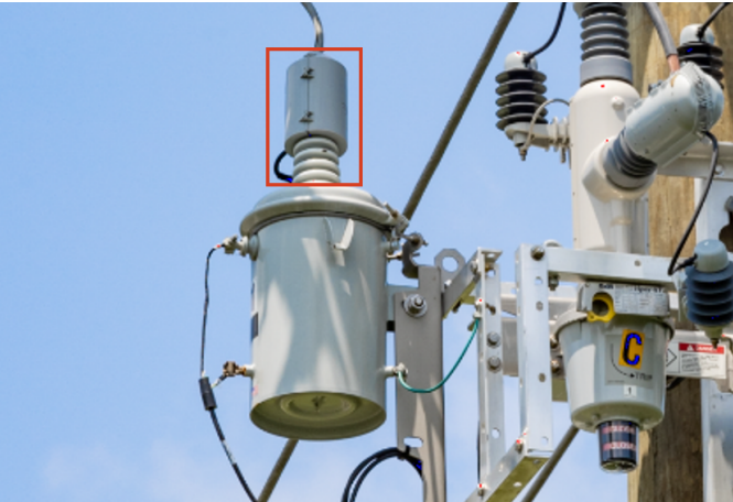
Fig. 2. Jumper termination hidden by animal guard.
