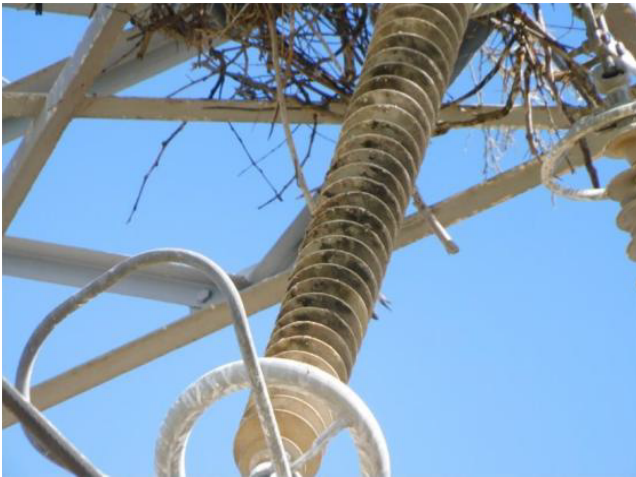
Fig. 8. Evidence found of the December 17, 2019, fault, showing bird contamination and arcing across the insulators.
