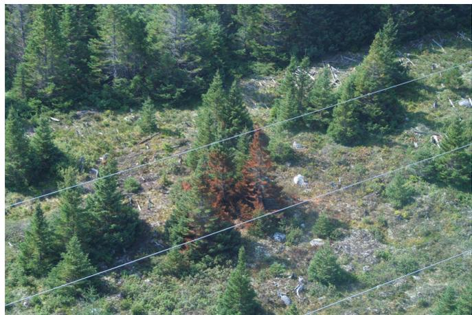
**Figure 4** Tree burned by flashover from 230 kV line
