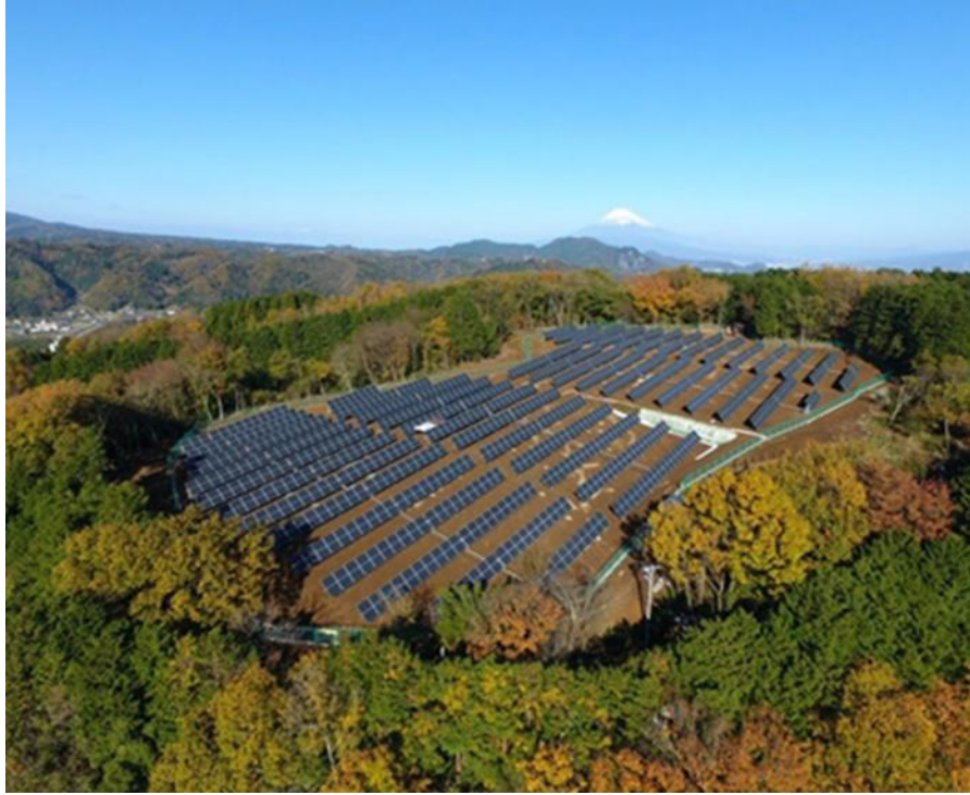
Figure 3 PV Power Plant
