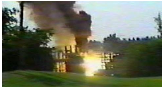
Fig. 1. Loss of a Substation Transformer After a DC System Failure
