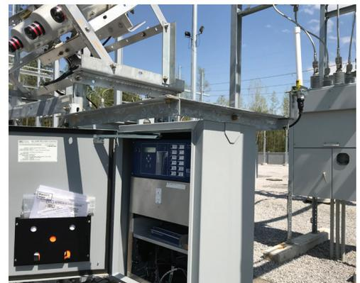
Figure 8—Omnidirectional antenna connected to SEL-FR12 to communicate with SEL-FT50 transmitters.
