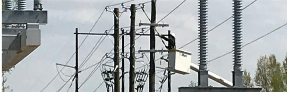
Figure 9—A line worker installs an SEL-FT50 outside the Northside substation on the overhead section of the feeder.
