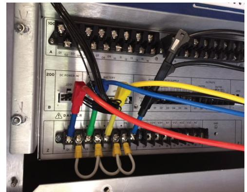
Figure 5—CT wired to SEL-651R current inputs in the test lab.
