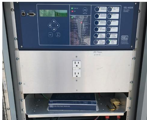
Figure 7—SEL-FR12 installed in the SEL-651R recloser control cabinet.
