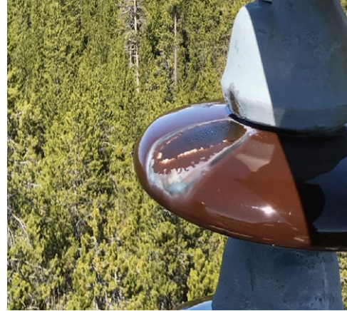
SEL traveling-wave fault-locating technology has a decade-long track record of accuracy on the order of one tower span.
