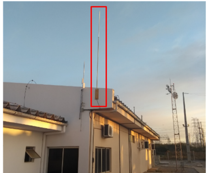
Fig. 4. Sensor installations on medium-voltage lines (left) and receiver antenna in the Brazil substation (right)
