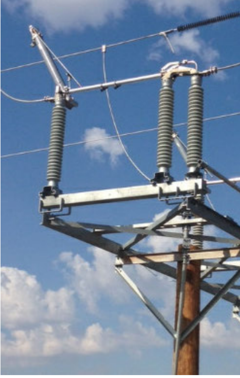
Fig. 2. Typical load-break disconnect switch.
