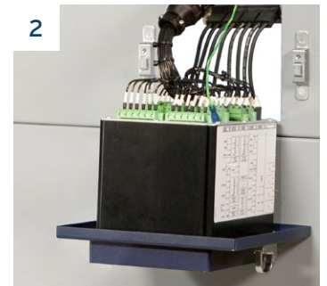
2 Hinge meter down.
