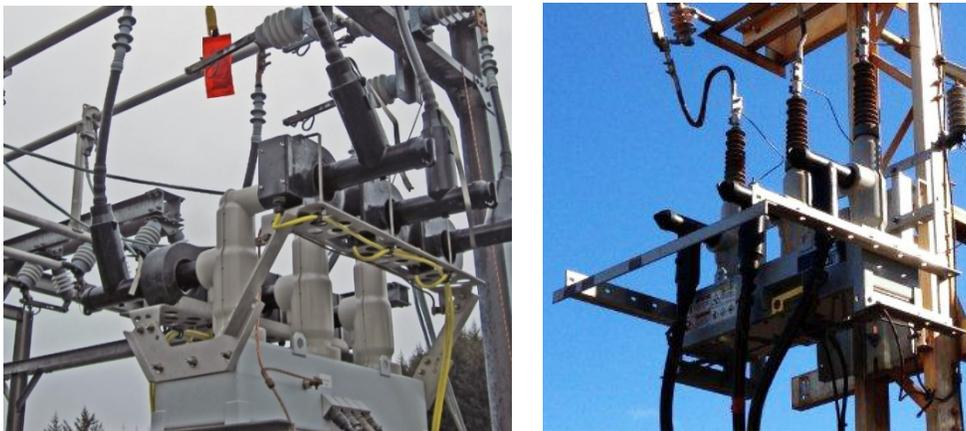
**Figure 11 Elbow-Connected G&W Viper Reclosers**
