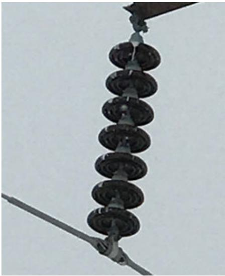
Fig. 27. Bird-contaminated insulator 16.395 mi from Drummond
