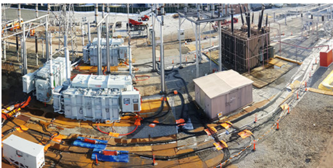
Fig. 1. Mobile Resiliency Transformers Deployed to Replace a 328 MVA, 345/138 kV Autotransformer
