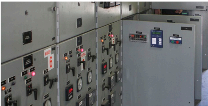
In many upgrades, just 1 or 2 digital relays can replace 20 or more EM relays and provide better protection.
