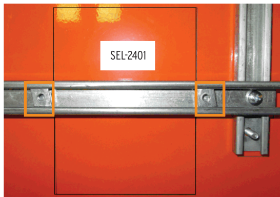
Figure 7 Install Channel Nuts
