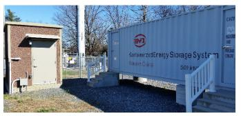
Fig. 14. Control House Exterior and BESS
