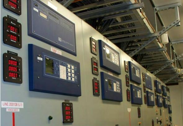
Fig. 1. Relays With Synchrophasors in Protection Panels
