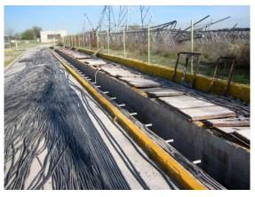
Figure 2 All These Copper Conductors Were Replaced With a Handful of Fiber-Optic Cables
