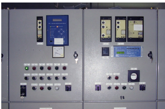
Figure 4—For an economical, high-speed retrofit, MOH abandoned the existing protection and metering, and installed new SEL relays in the switchgear.
