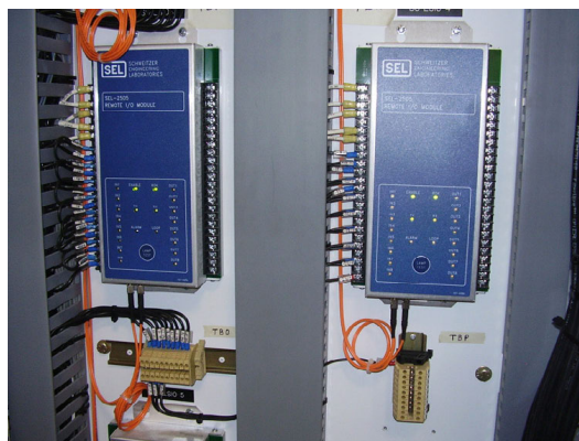
Figure 6—Ultrahigh-speed, remote-mounted I/O modules were installed throughout the plant for the SEL POWERMAX load-shedding system. These control (DIP) switch-configured I/O modules have trip-rated output contacts, devoted communications, on-board power supplies, and full self-monitoring for the utmost reliability.
