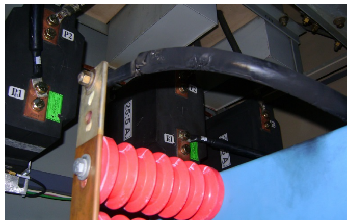
Fig. 30. Fast tripping for a cable failure at the generator bus limited its damage; the cable repair cost was minimal.
