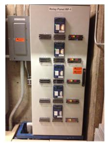
Figure 3. Melt shop switchgear relay panel (with complete protection for five circuits)
