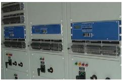
Figure 3. Microprocessor-based relay panel
