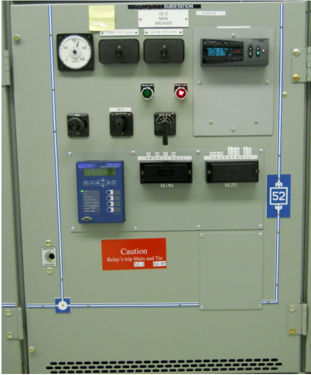
Fig. 9. Switchgear Breaker, Relay, and Controls
