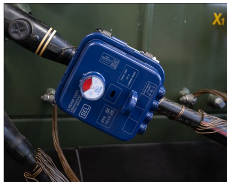
A UGFI provides fault indication inside pad-mounted switchgear or underground vaults.
