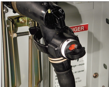
A TPR with junction shield provides fault indication inside switchgear.
