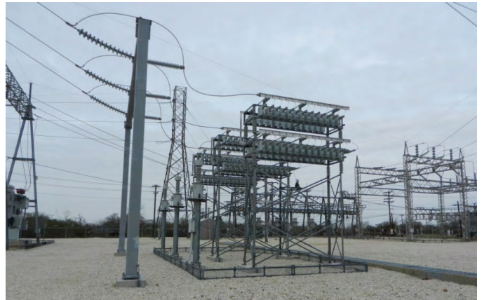
Fig. 1. 31.2 MVAR shunt capacitor bank at 138 kV substation.
