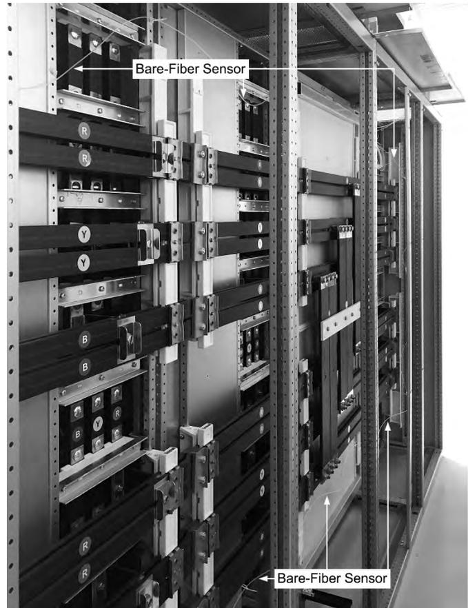
Fig. 14. Bare-Fiber Sensor Around Busbar Perimeter of 415 V Switchboard
