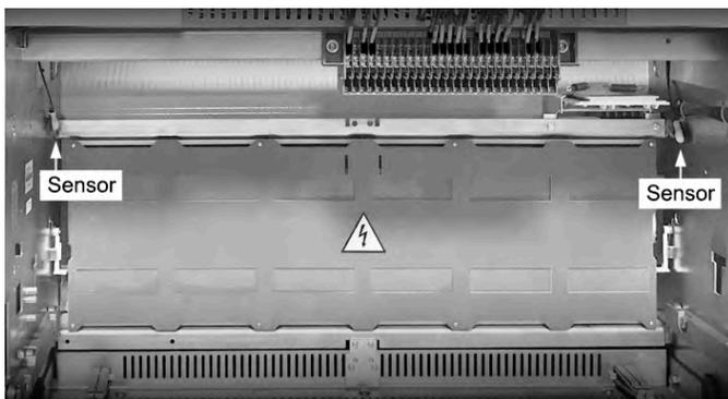
Fig. 13. Point Sensors in Breaker Compartment of 415 V Switchboard
