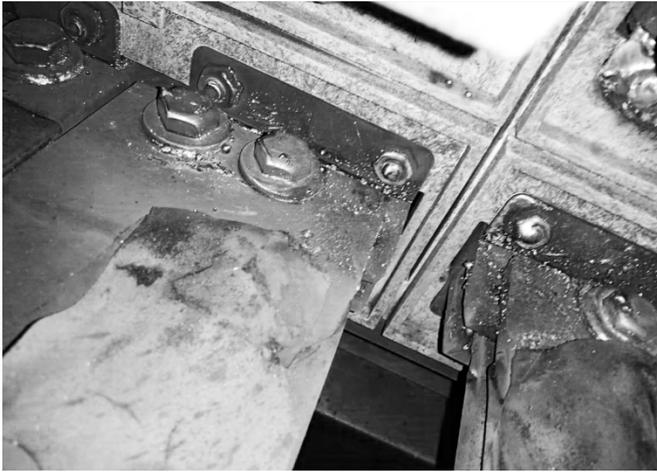
Fig. 20. Fault Location at Breaker Output Terminal
